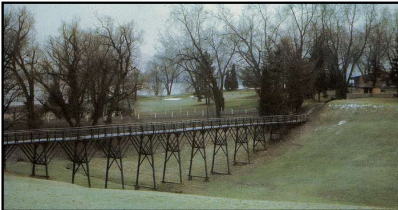
Bridge on Hole #1
