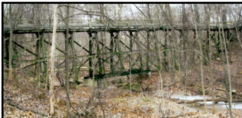
The Only Large Remaining Bridge
